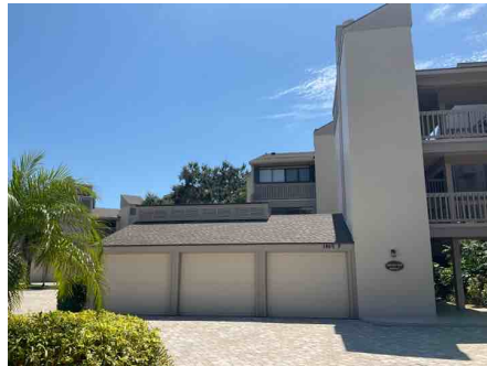
Elevation and unprotected glazed openings
