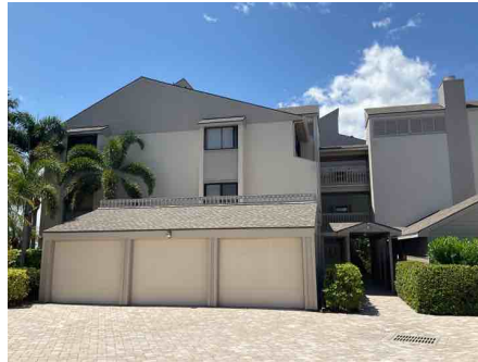
Elevation and unprotected glazed openings
